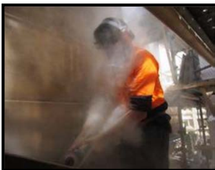
Figure 4: ‘Chopping out’ no dust shroud Source K. Alamango 2015
