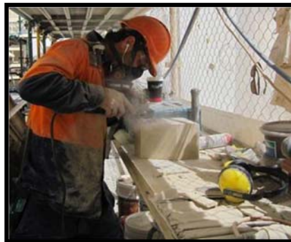
Figure 2: ‘Spinning’ with angle grinder
