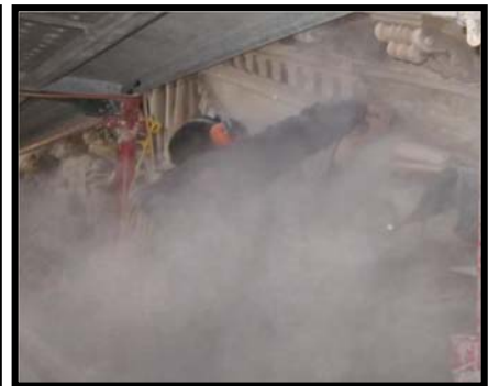
Figure 3: ‘Chopping out’ with grinder
