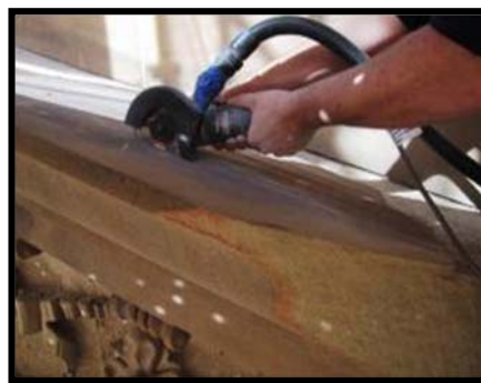
Figure 5: ‘Chopping out’ with dust shroud
